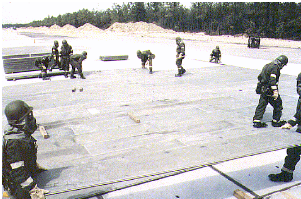
Figure 5.3. AM-2 Mat Repair Method.
