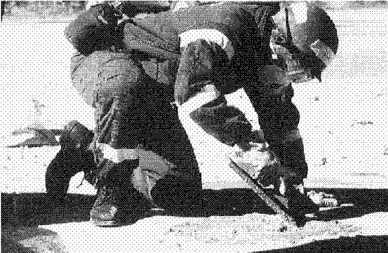
Figure 5.49. Leveling Silikal®.
