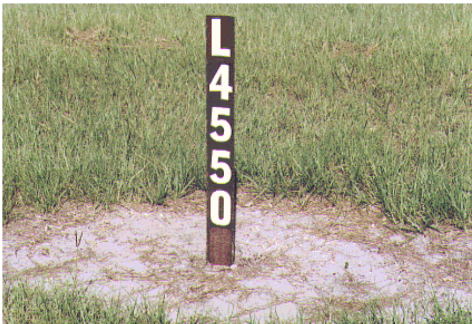
Figure 5.26. Raised Pavement Marker System Post.
