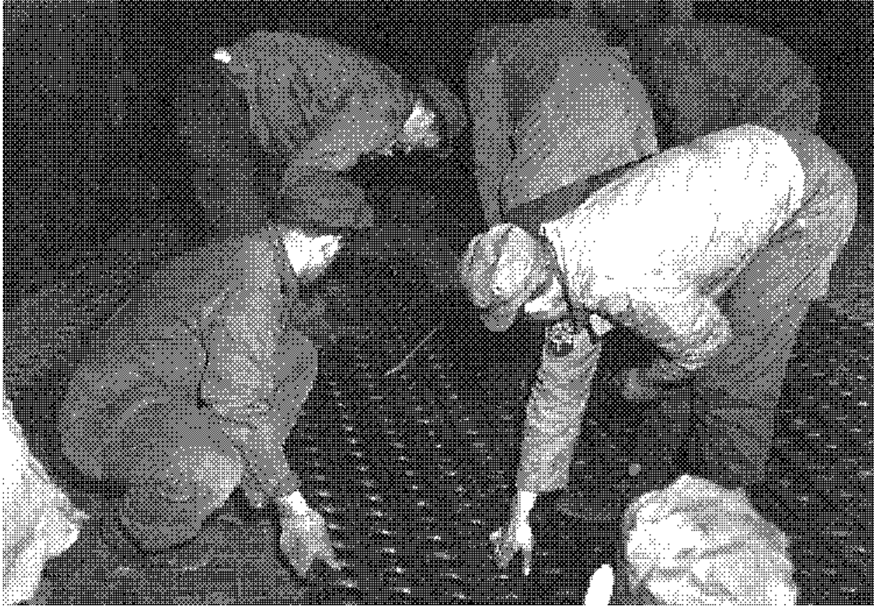
Figure 1.1. PSP Being Installed at Night by Men of the IX Engineer Command at an Air Base in Germany in 1945.
