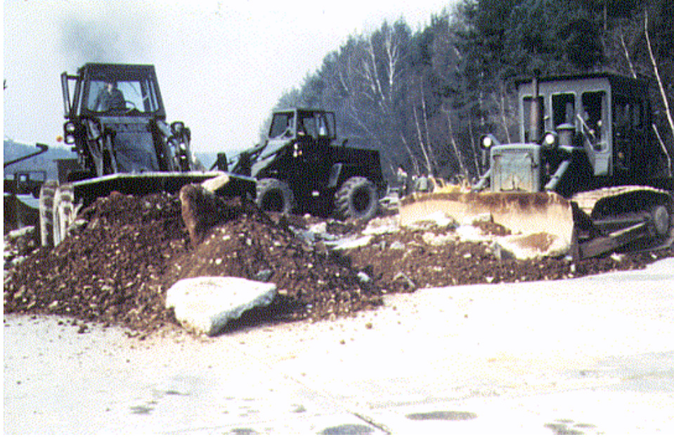
Figure 5.23. Upheaval Removal.
